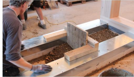
Decken Rahmen "Schalung"
